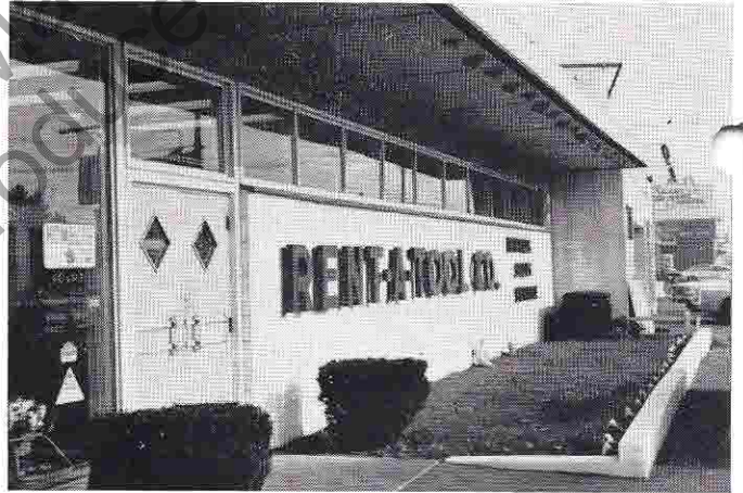
The trim exterior of Rent-A-Tool Co. stands out like a beacon on busy Route 22 in New Jersey. A fine, large neon sign dominates the whole area.
