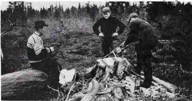
A three man team and one small XL-12 pile up an impressive cutting record in Finland.
