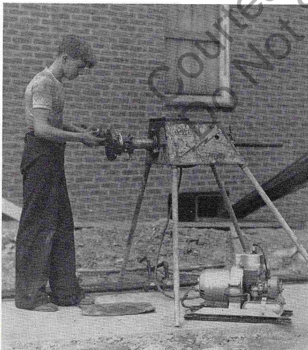
Speeding pipe threading for a plumber
