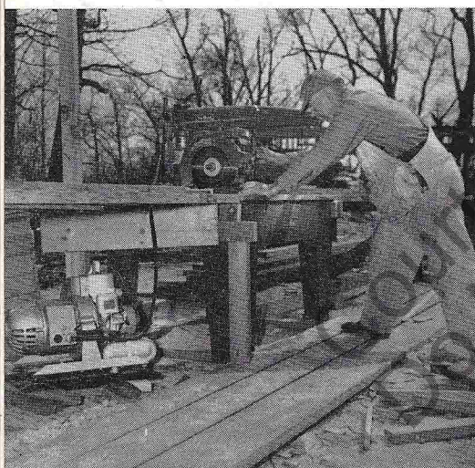
Operating a saw for industrial building
