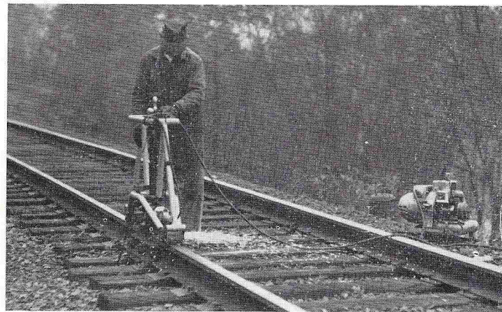
Running a grinder on railroad tracks
