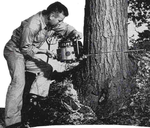
Clearing trees for a construction site
