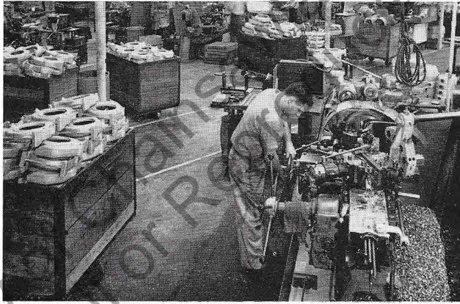
One of the many turret lathes in the machine shop
