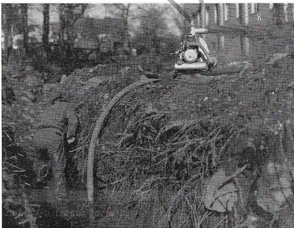
Pumping a trench for a sewer line
